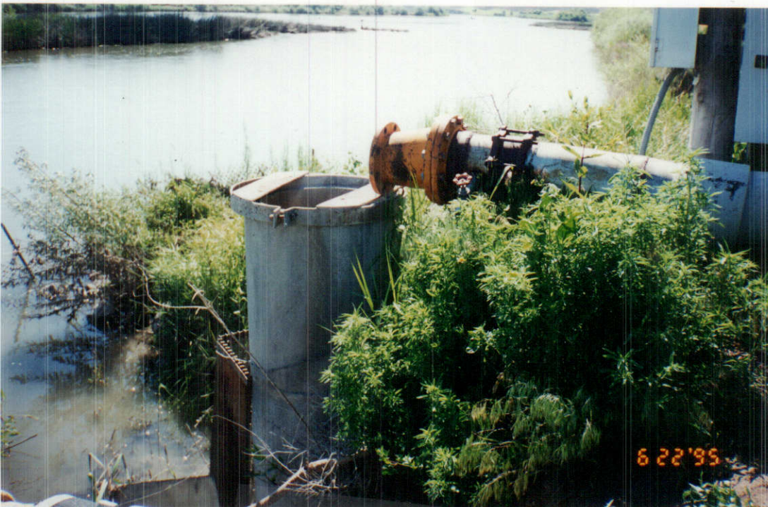
← Gravity System (pump out for repairs)
