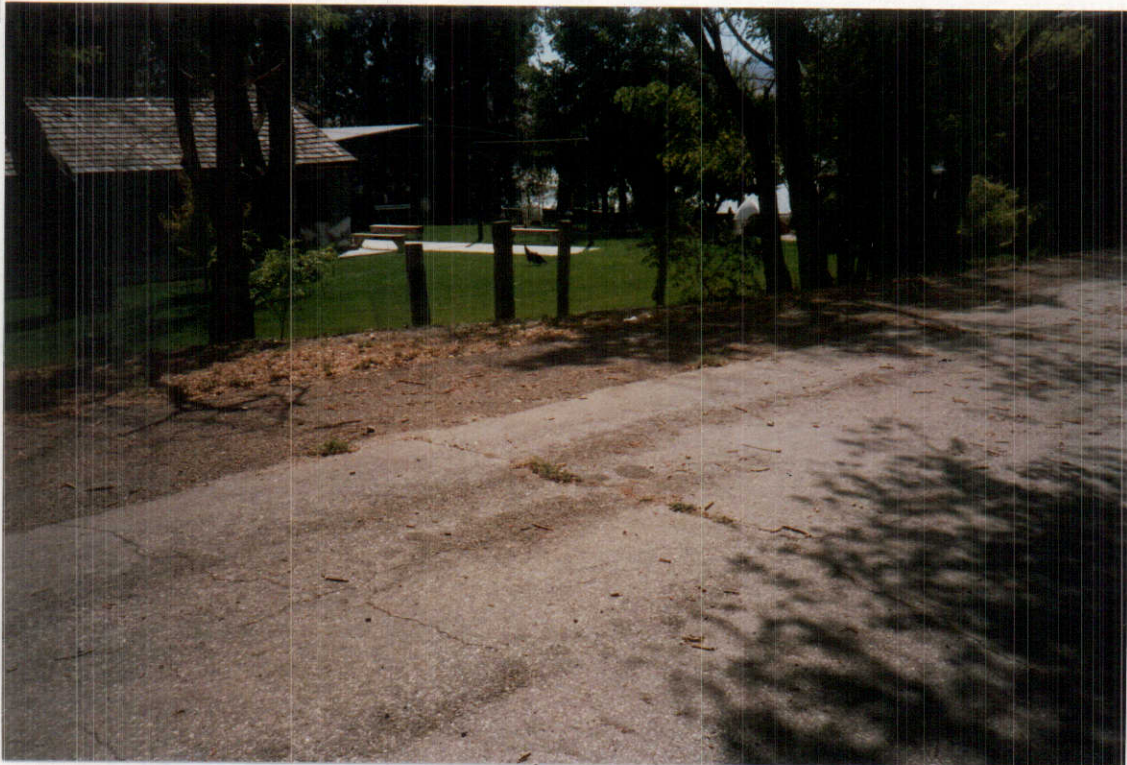
Place of use - Museum & surrounding Area Walters Ferry Bridge
