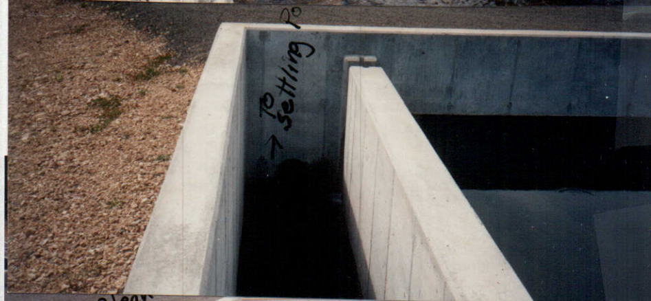
Clean Out Pond
