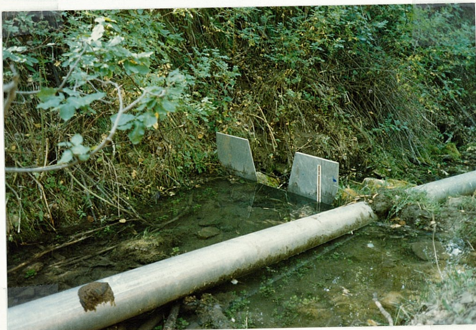
Cippolatti weir (Badger meter is downstream just 20 or 30' on mainline)
