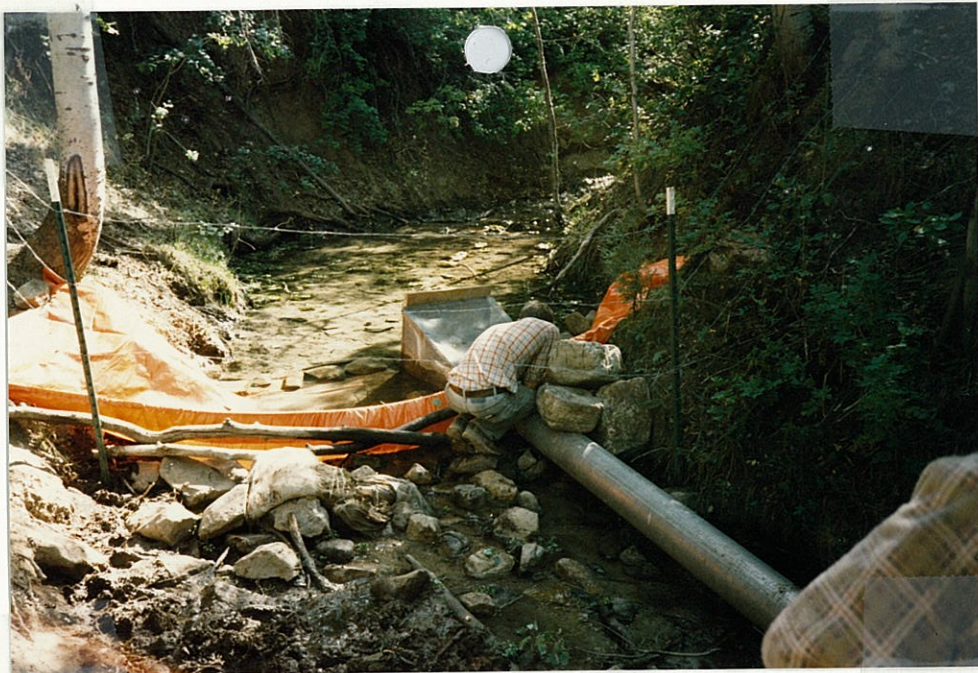
Dam on spring
