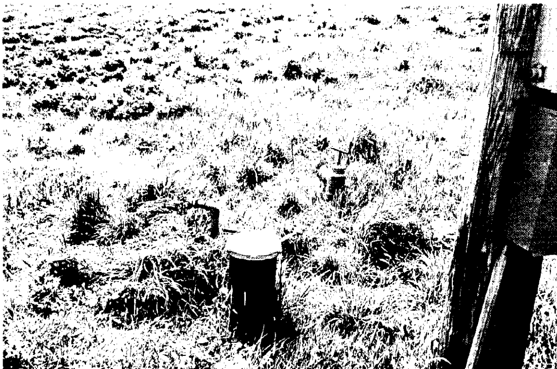
3. and 4. Well with crop and handline in background. Well pump connected to mainline and handline risers.
