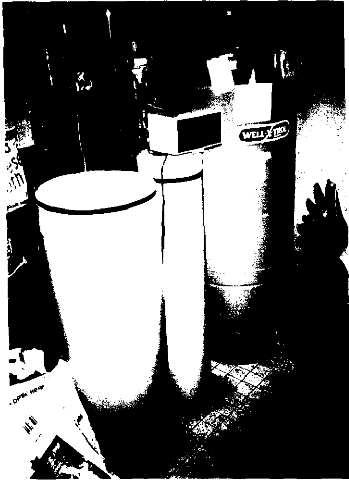
Pressure Tank and water Soft, hooking East
