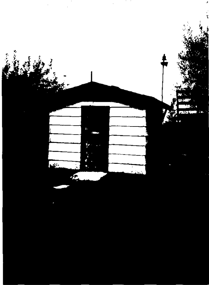
Plate 1 - Pumphouse at point of diversion.
