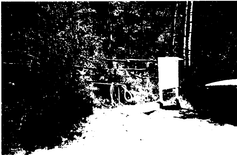
HYDRANT BY ROAD, WITH FIRE HOSE.
