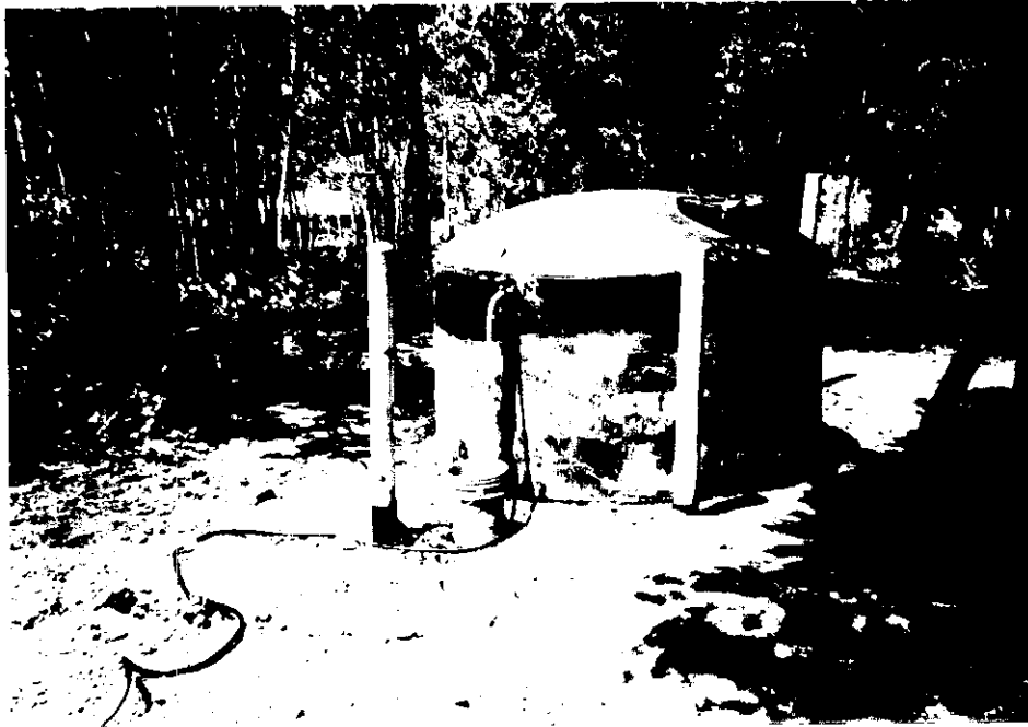
1300 GALL. TANK FOR STORING WATER.
