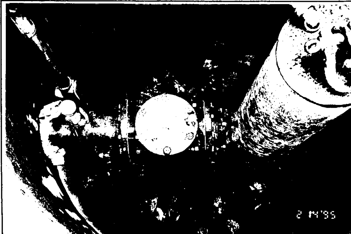
PICTURE OF 10" WELL, CHECK VALVE AND PRESSURE GAGE.
