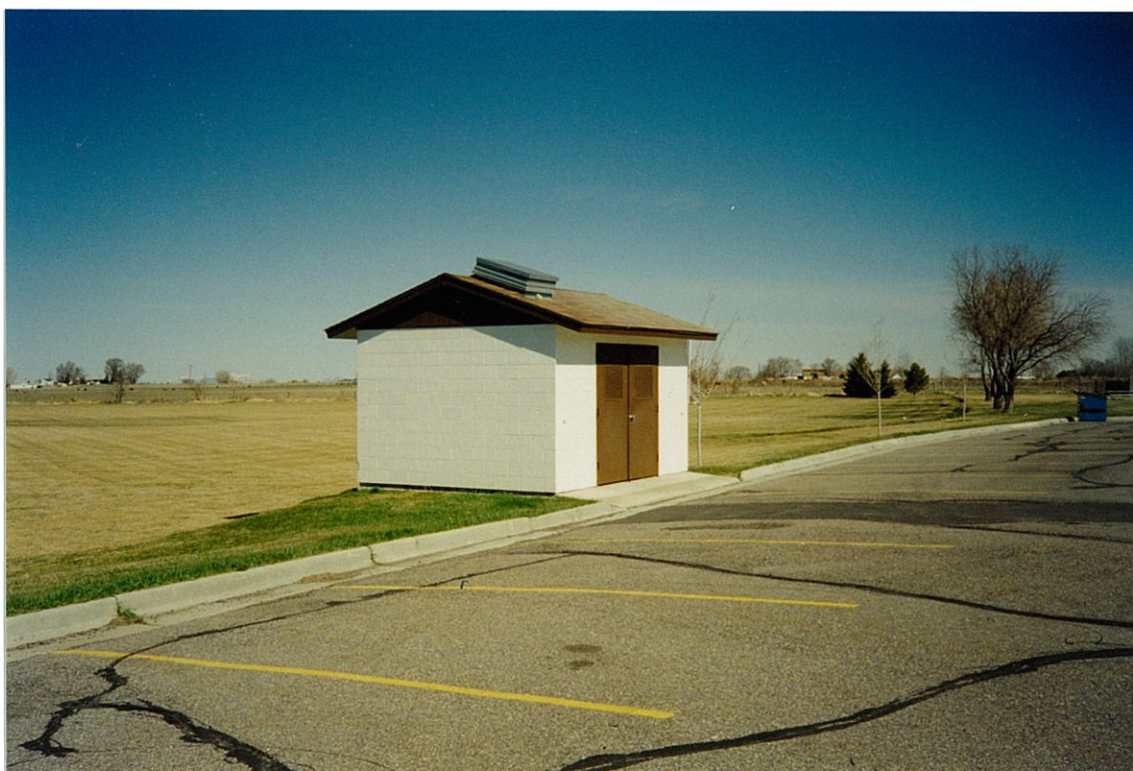
Plate 1 - Pumphouse at point of diversion for irrigation of playfield.
