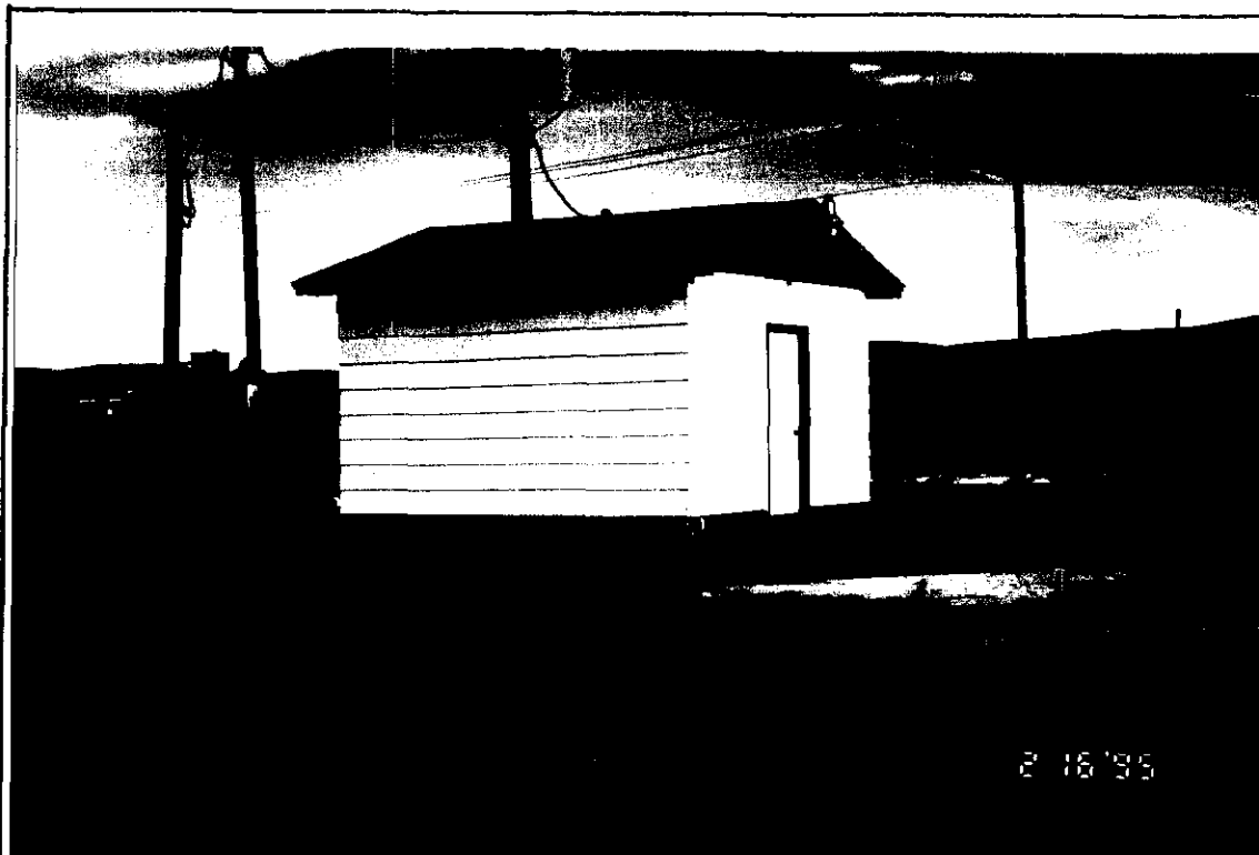
VIEW OF PUMP HOUSE
