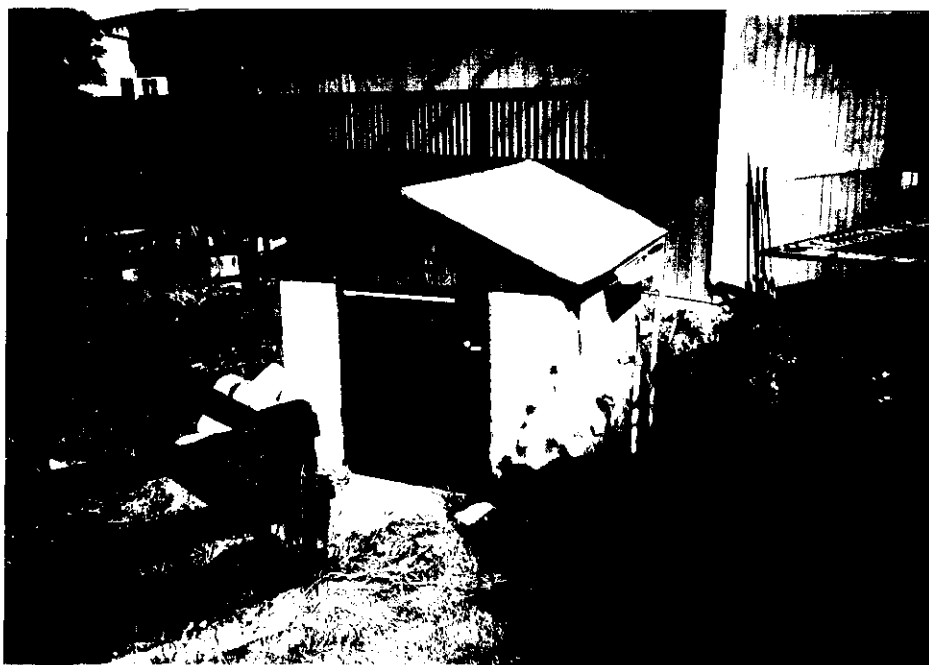
Plate 4 - Closeup of pumphouse.
