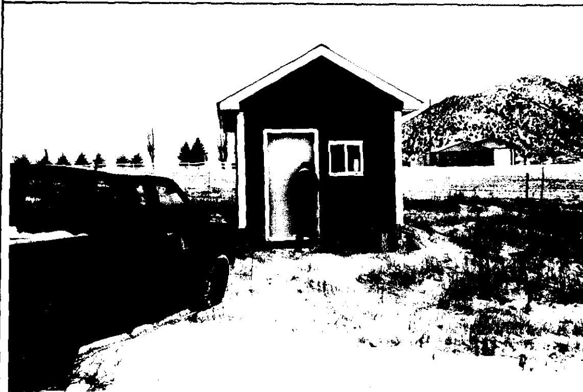
WELL AND CONTROL HOUSE
