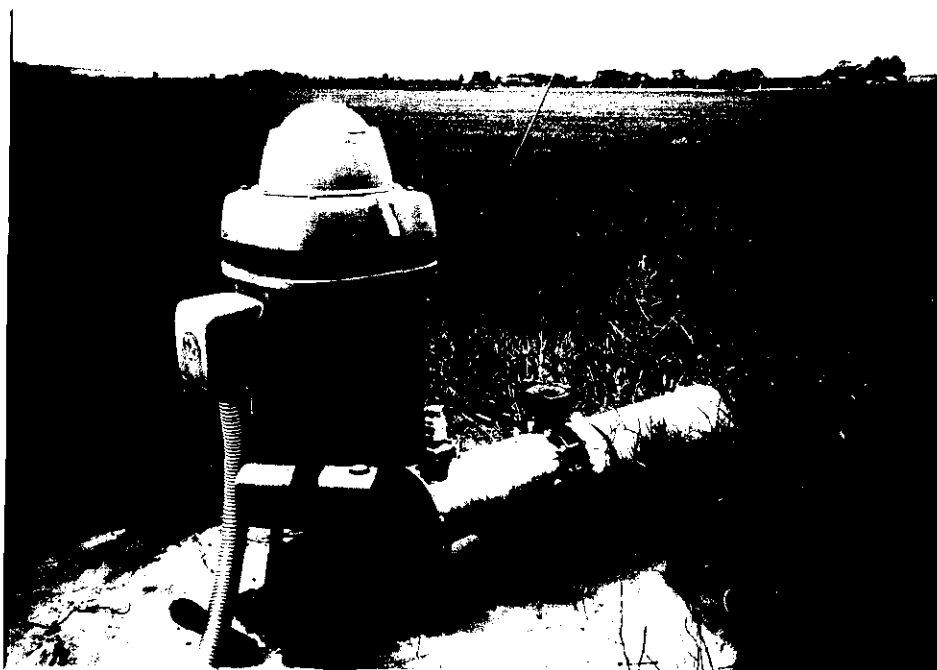
Fig. 2 - Point of diversion looking southwest.
