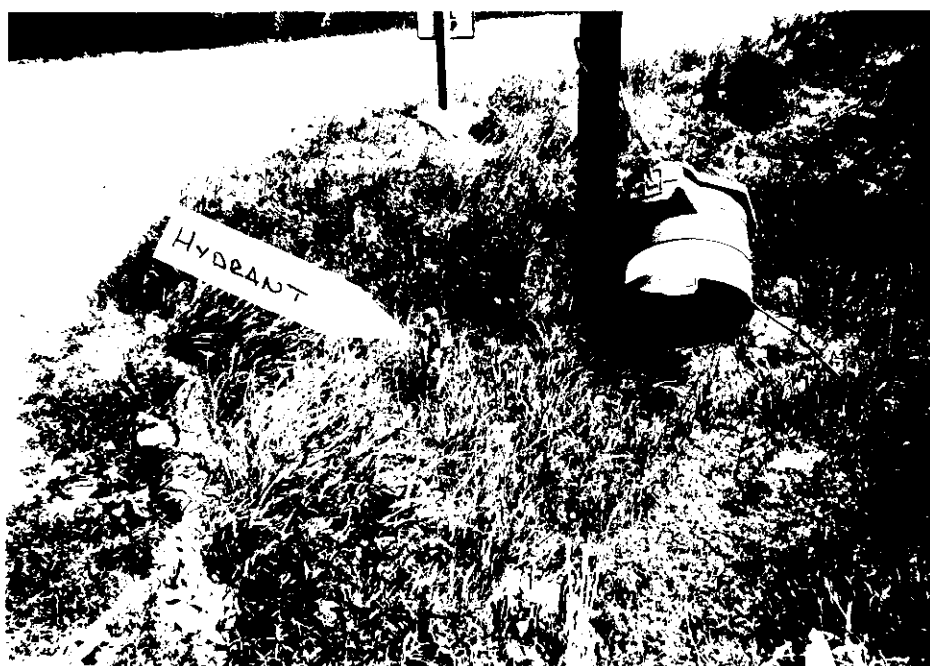
Fig. 2 - Hydrant at entrance to landfill.
