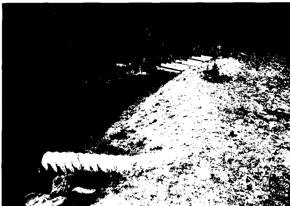
Plate 4 - Overflow culverts (upstream side of dam).
