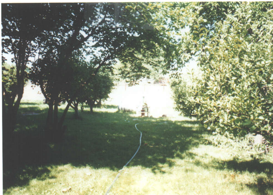
-PIPE LEADING TO HOUSE FROM WELL
