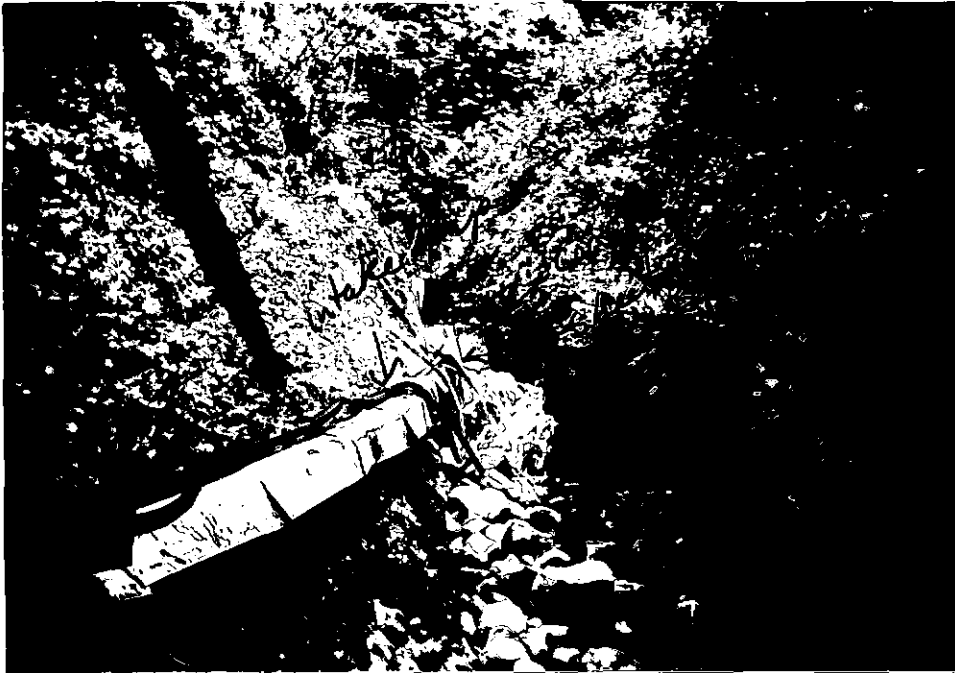
Point of Diversion
