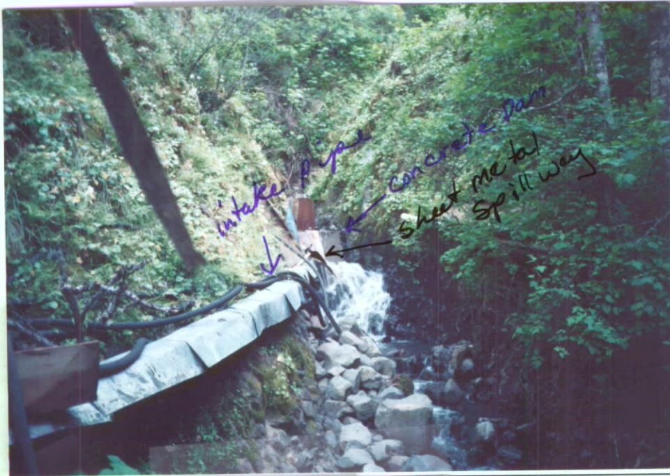
Point of Diversion
