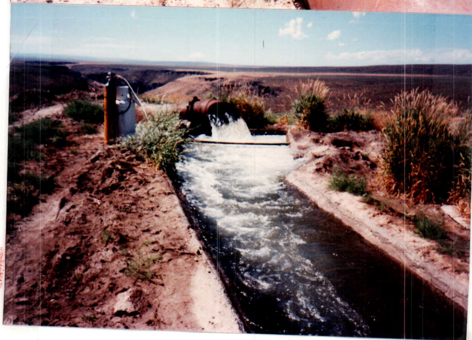
Discharge into ditch
