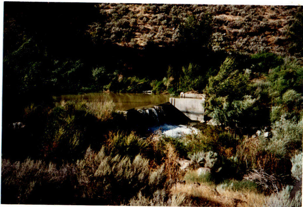
Diversion Works. Concrete structure feeds pipeline.
