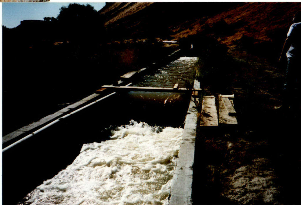
Outlet of pipeline to concrete measuring device.
