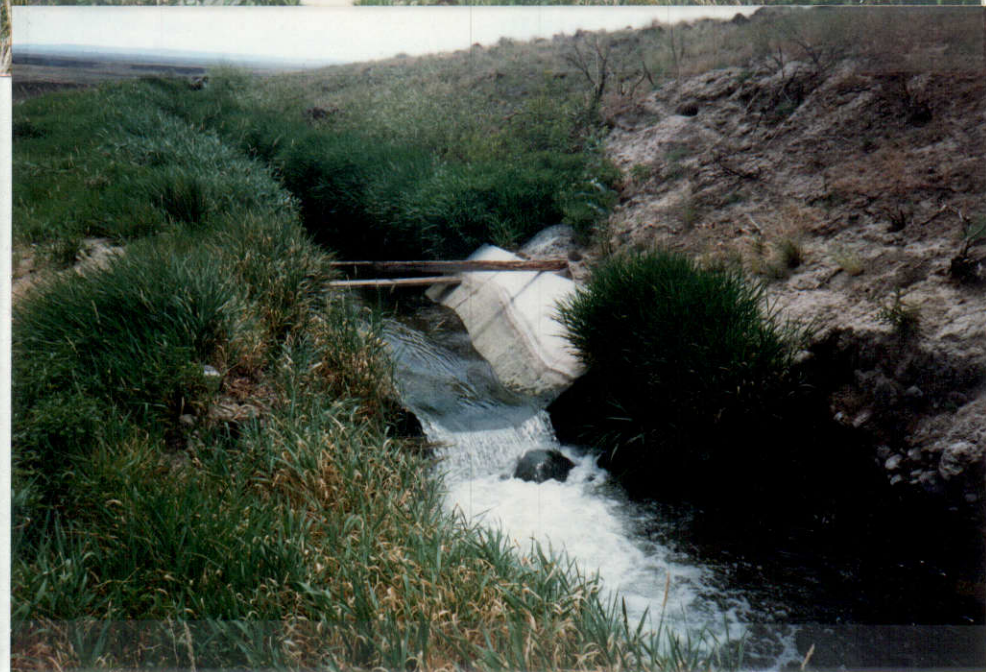
#2 Trapezoidal weir at head of Marshall - Easterday canal. Output from pumping plant on Salmon Falls Creek measured here.
