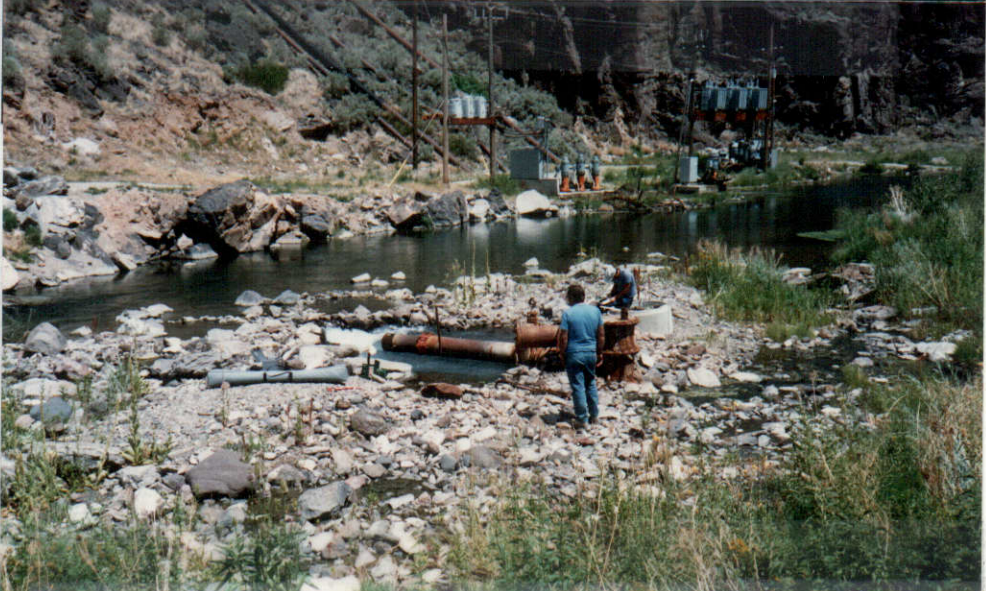
Marshall's Well in foreground with Wright's pumping plant & Marshall - Easterday pumping plant in background.
