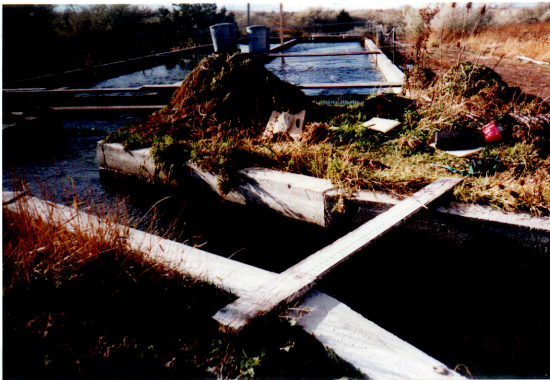
Measuring Point - Parallel Channel Section
