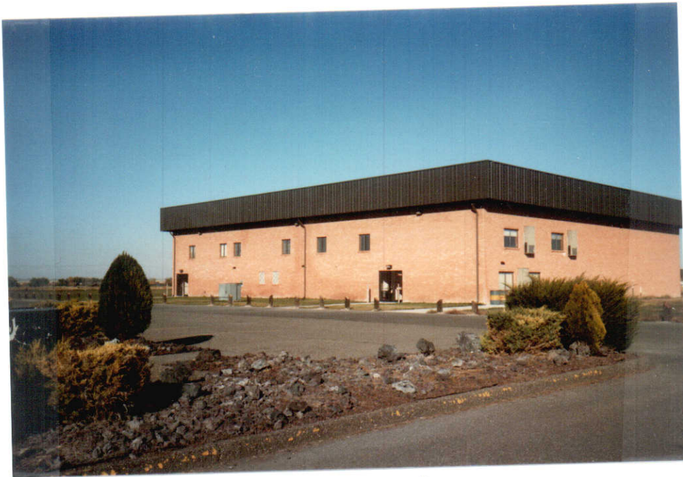
Multi Purpose building
