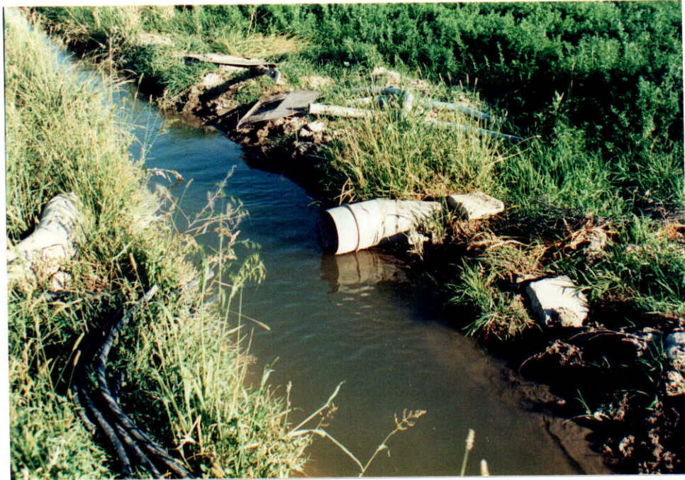
Photograph #3 Discharge into existing surface ditch.
