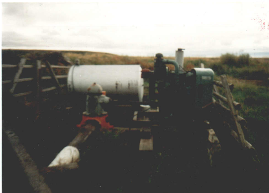
P.D. Looking west
