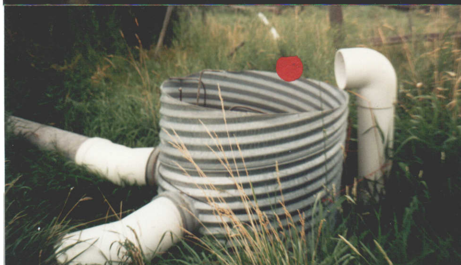
Stand Pipe Looking N.W. To P.O.
