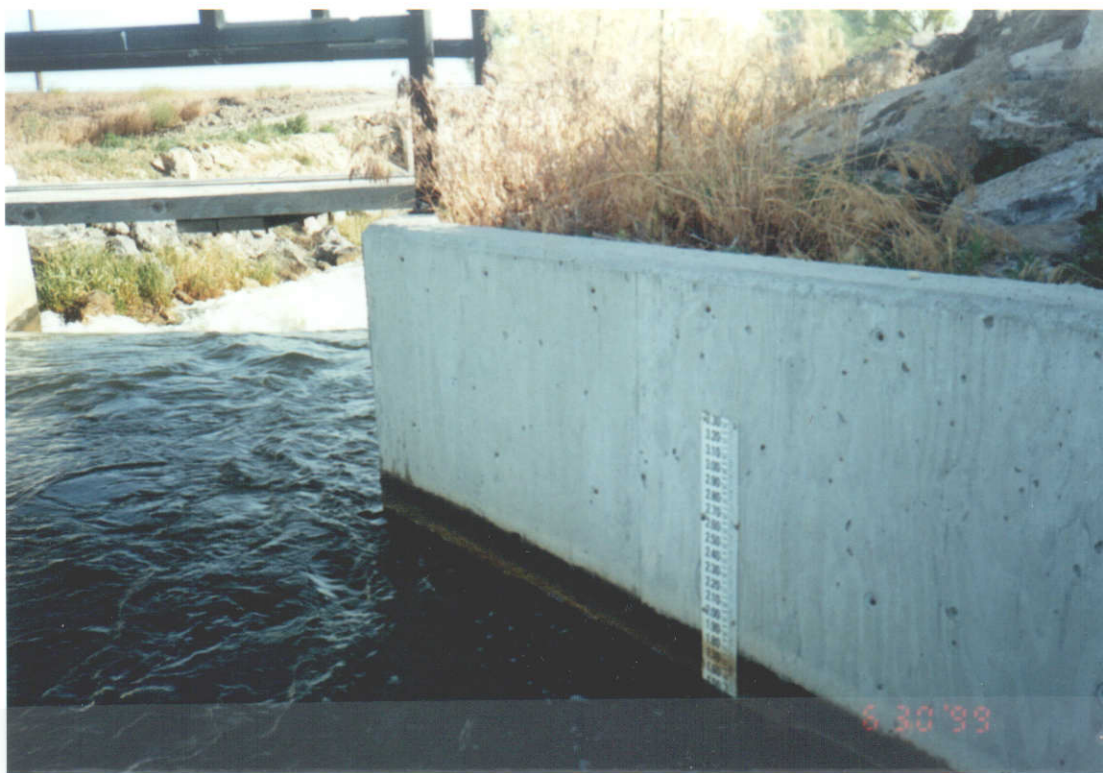
Staff Gauge at TFC Weir
