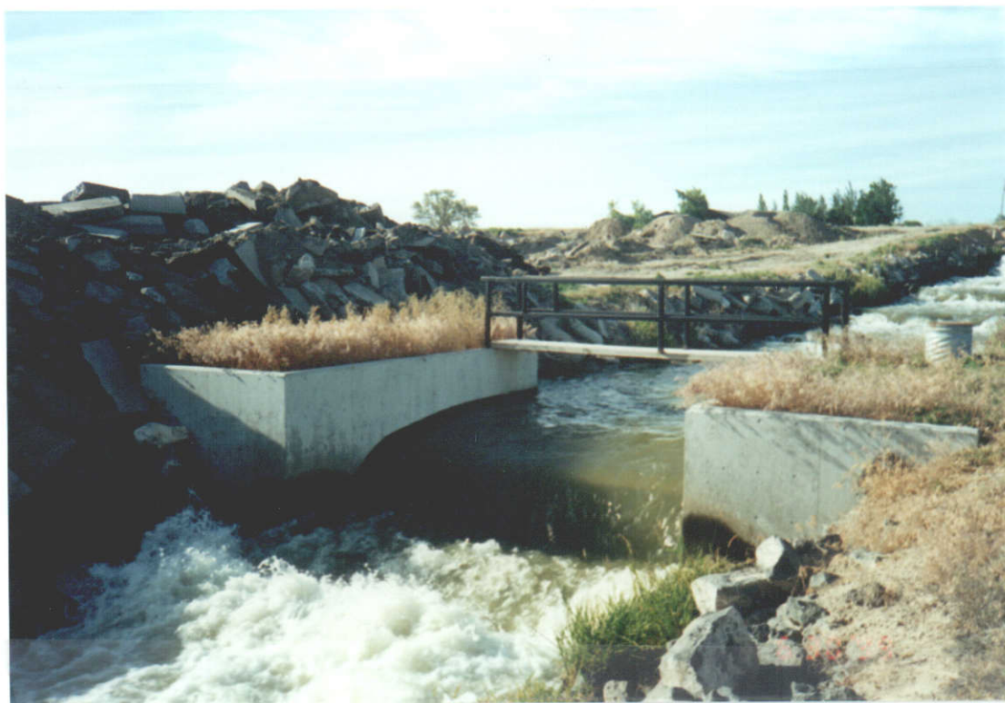
Downstream (North) End of Weir
