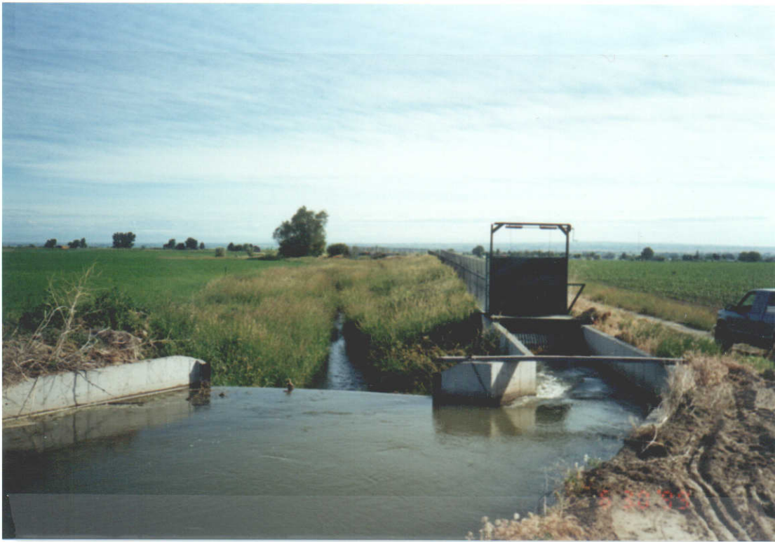
Conlee + Head of Penstock (Looking North)
