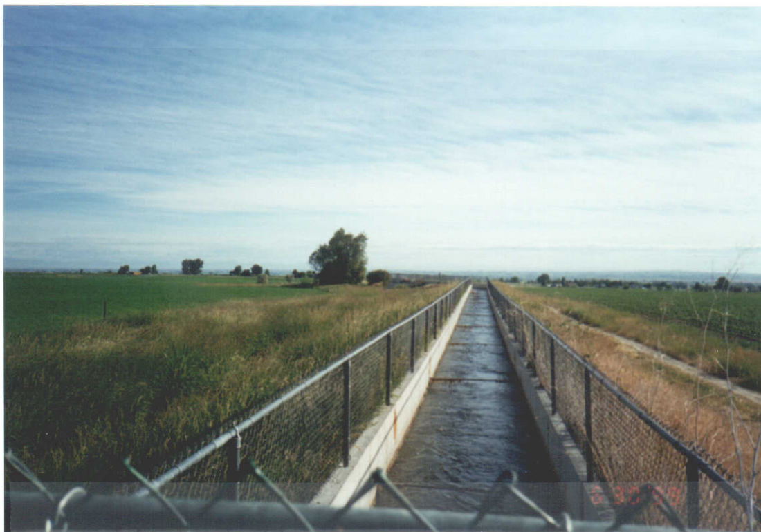
Penstock (Looking North)
