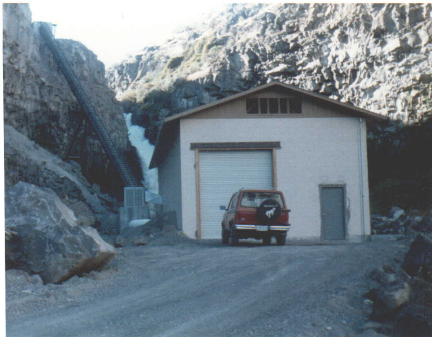
Powerhouse And Penstock Looking Upstream
