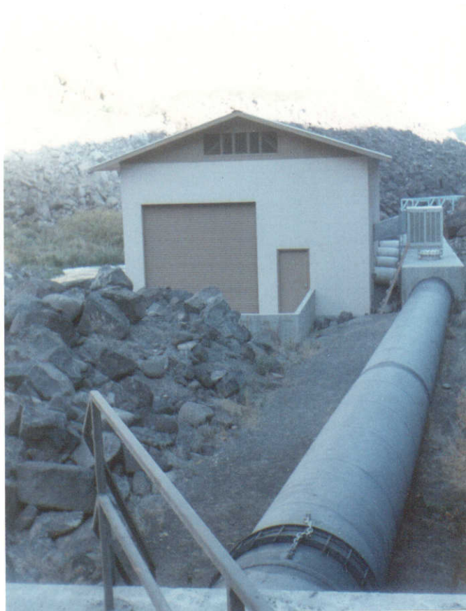
Powerhouse And Penstock Looking Downstream
