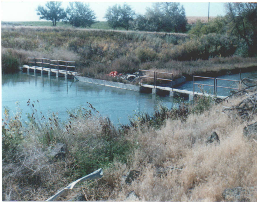
Diversion on Cedar Draw Creek (Looking Downstream) Cedar Draw Creek Branches To Left, Power Canal To Right.
