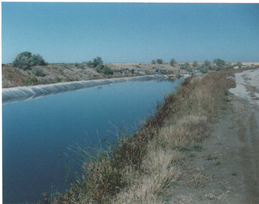
Power Canal With Penstock Intake Structure In Background. (Looking Downstream)
