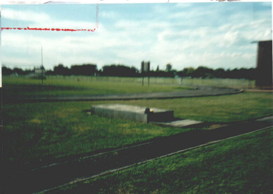
Concrete structure well house
