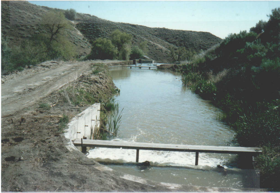
Upper pond used at present as settling pond
