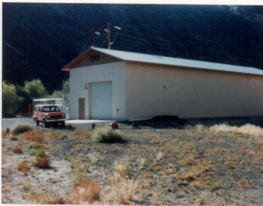
CRYSTAL SPRINGS HYDROELECTRIC PROJECT POWERHOUSE
