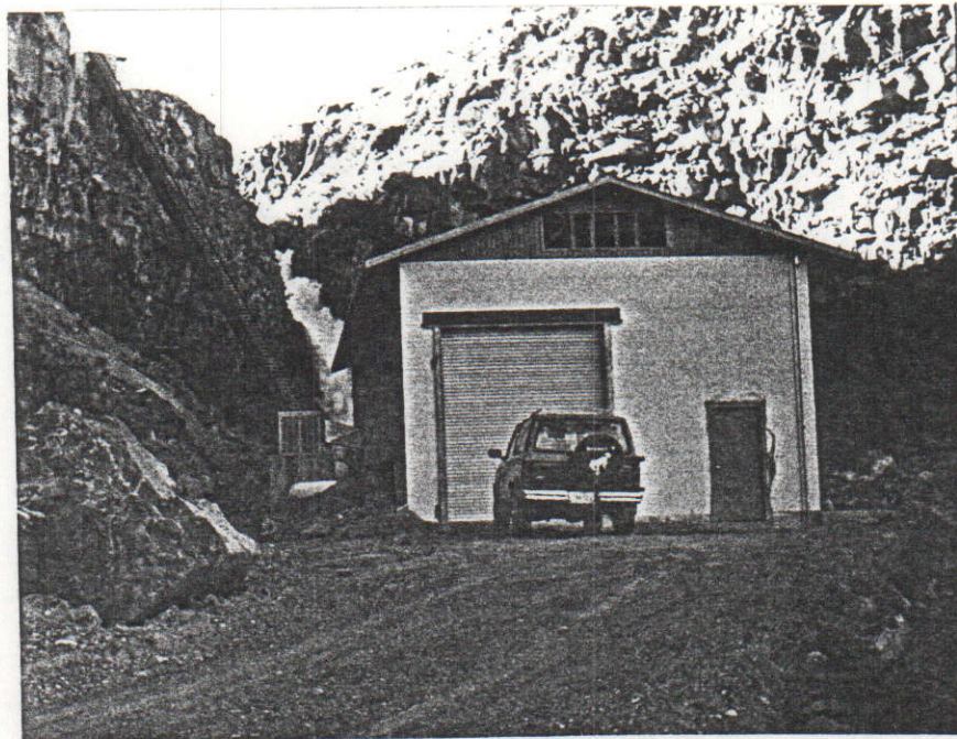
Powerhouse And Penstock Looking Upstream
