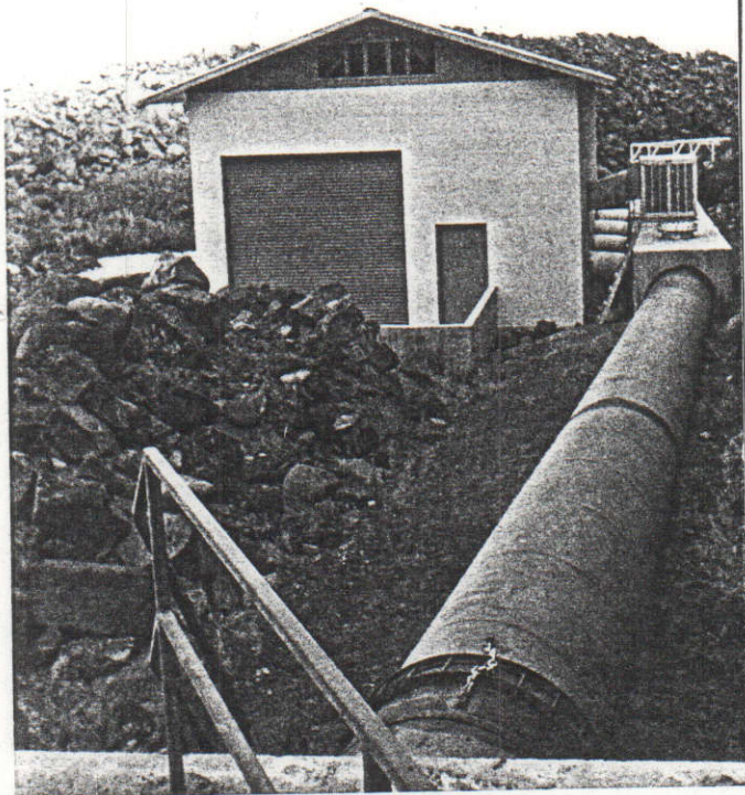
Powerhouse And Penstock Looking Downstream
