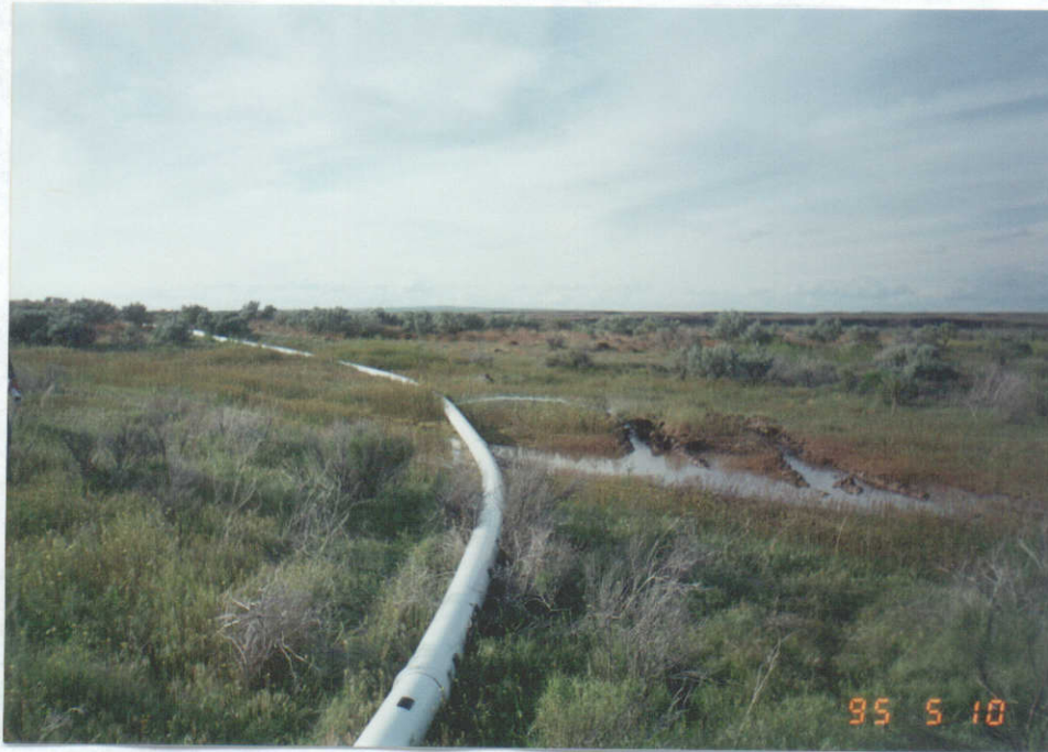
Figure 5 Stutzman 47-08019 Gated Pipe Distribution System
