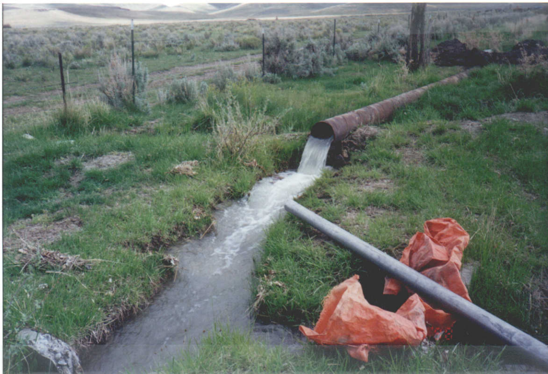
Cans/ Water Discharging From Steel Pipe. Aluminum Pipe From Well #2
