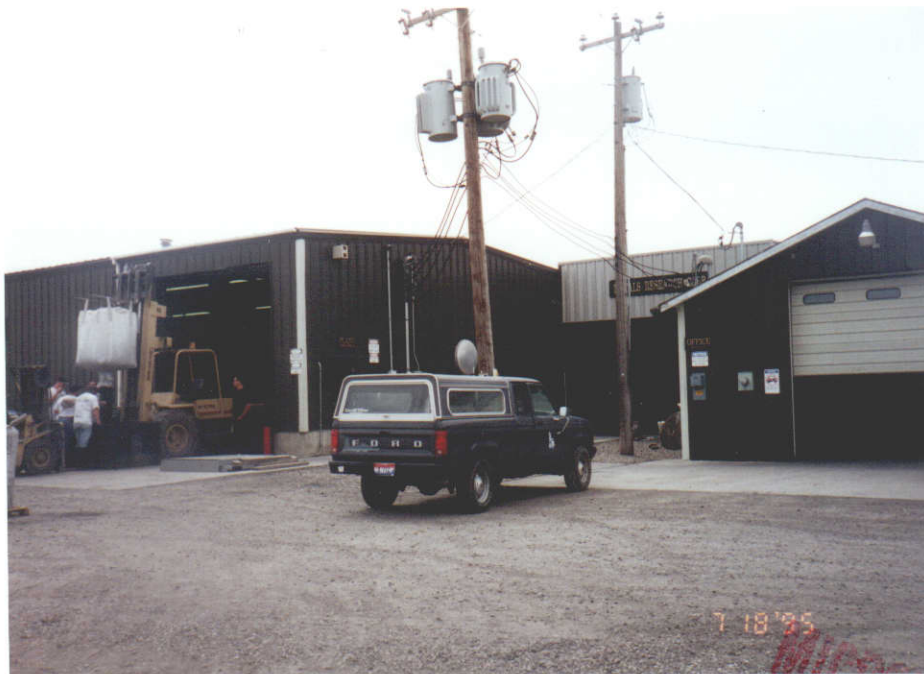
P/U #1 (Plant, offices, Laboratory & shop for well # 1)
