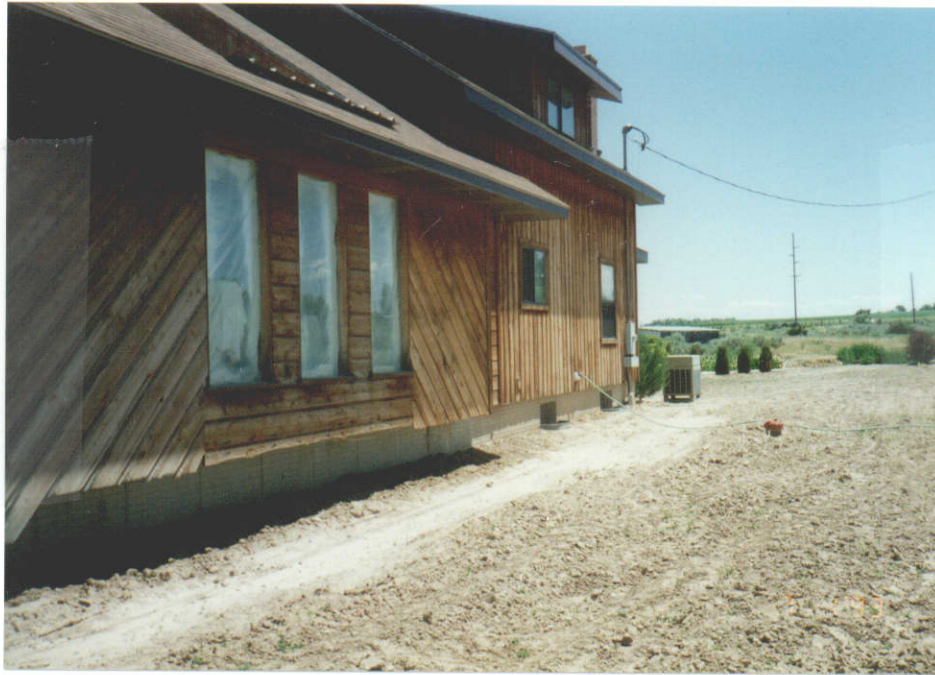
WEST WELL BEHIND HOUSE
