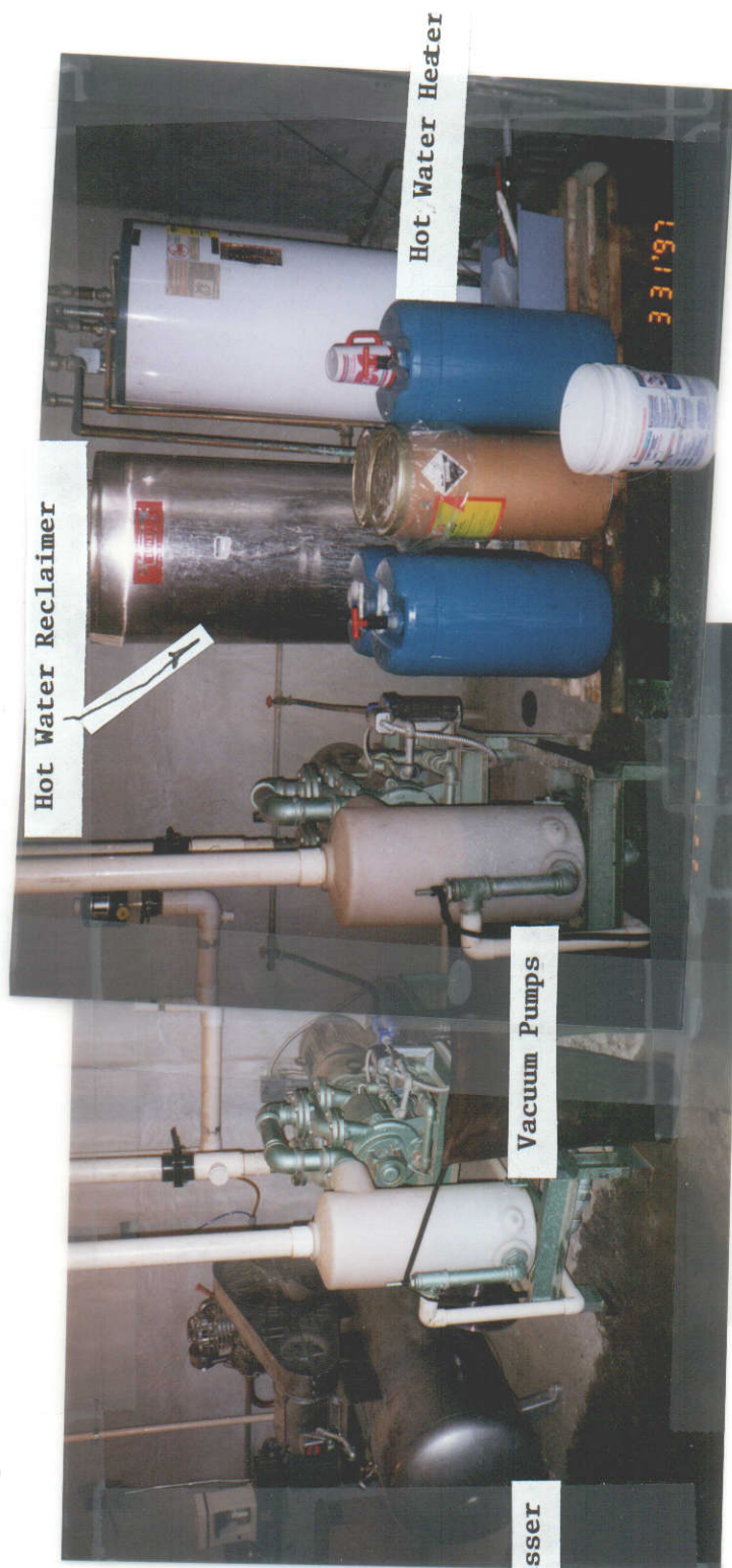
2 Pressure Tanks used inconjunction w/ 10,000 gallon holding tank
