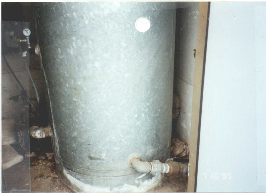
→ P.O.D 300 GAL Pressure TANK
