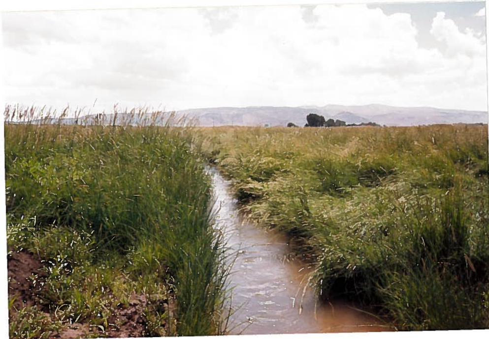
Looking south at ditch running to pond. Ditch approx 3' x 1' deep
