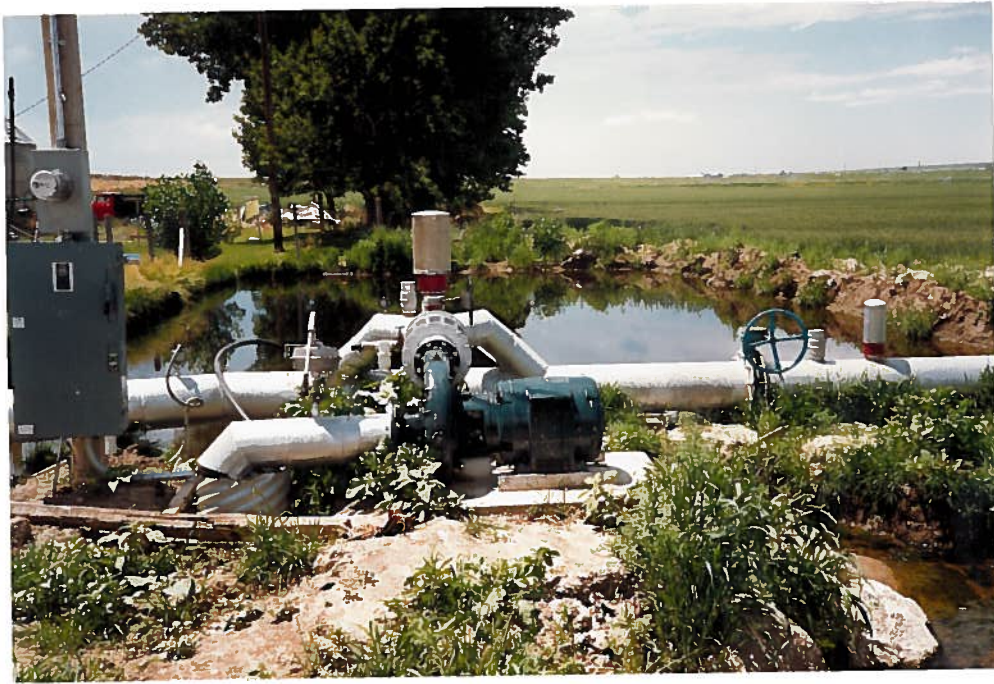
75-HP Pump and Pond, dry creek Decreed Rights . This system is Hooke Lin // with P/D
