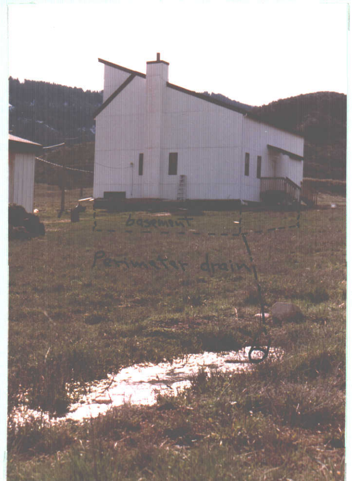
Figure F. Perimeter drain location and outlet.
