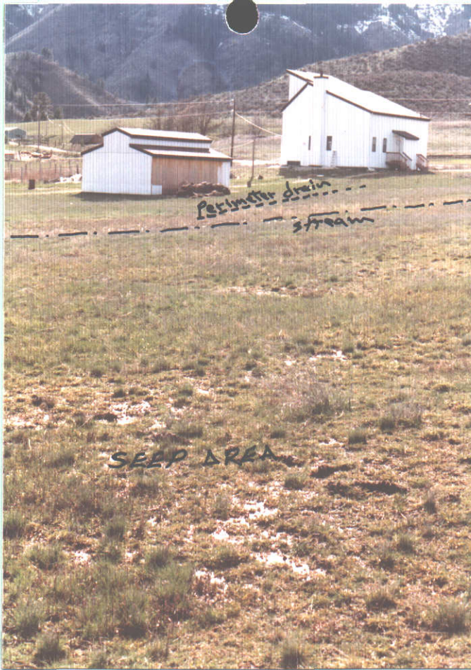
Figure E. Seep area and stream and perimeter drain location on subject lot.
