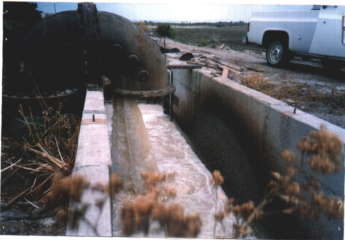
"Upper most" discharge point of the under- ground system. Located in the S.E. corner of the NE \frac{1}{4} of the NW \frac{1}{4} of sec. 20. Looking west.
