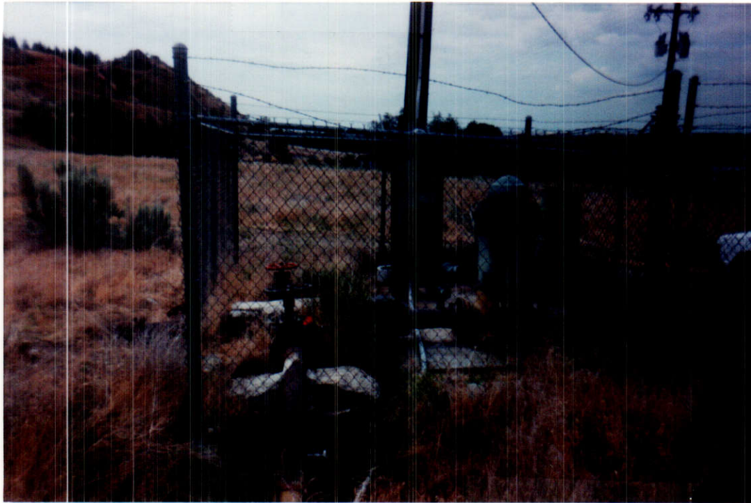
View of well : pipe to underground DISPERSMENT. Wall is headed toward the south of the P/U.
