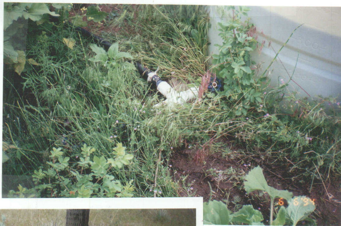
500 Gal storage tank, controlling works - 1
