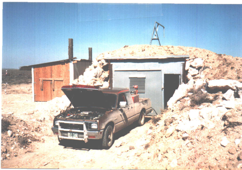
Pumphouse for Permit No. 63-10379
