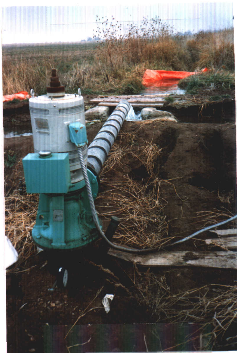
Kenneth Aschenbrenner - 63-10393 Diversion Facility
