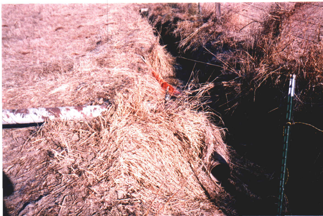
'T' section at point of discharge into ditch.
