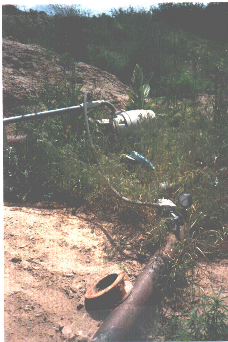
PICTURE # 4 RELIFT PUMP LOOKING EAST
