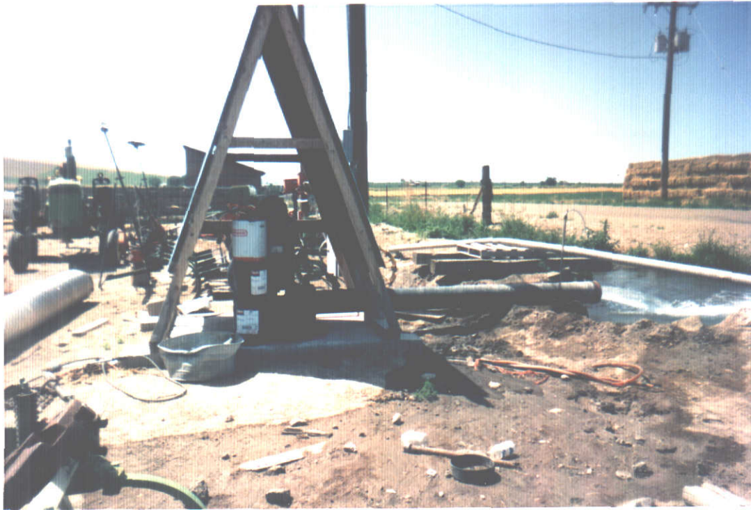
View of well. well has measuring device installed
