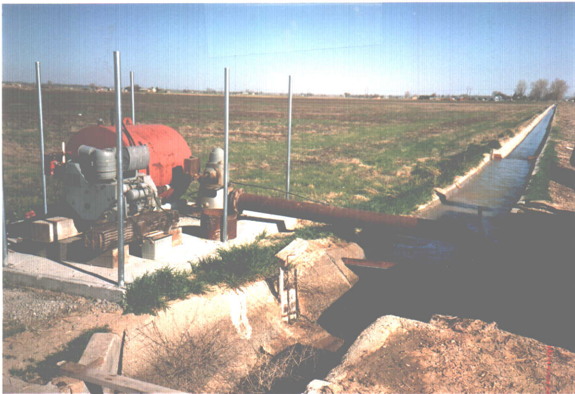
PHOTO TWO-Taken looking northwest shows the pump site, concrete ditch, part of the pou is in the background.
