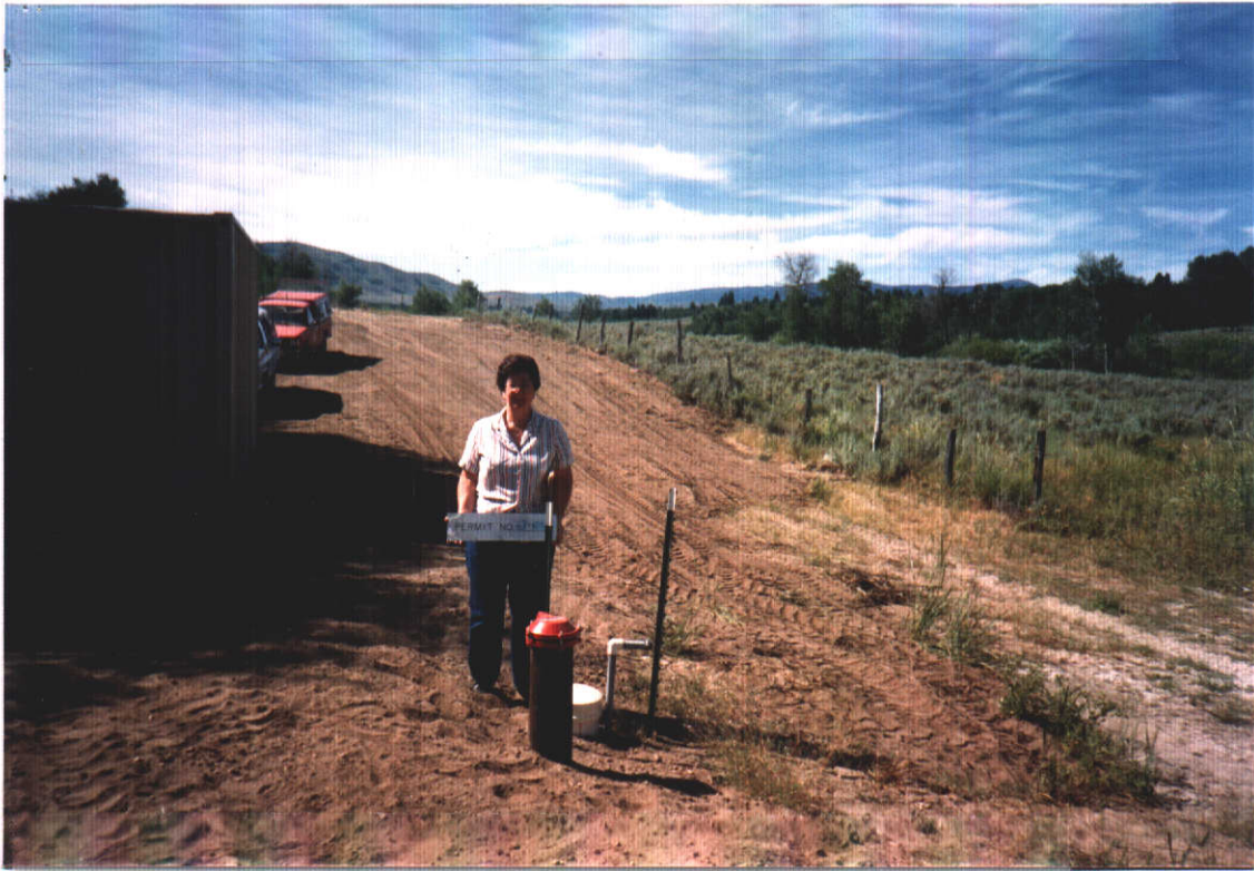
WELL SITE ON WEST SIDE OF LESTER CREEK ROAD ON RIGHT OF WAY LAND.
