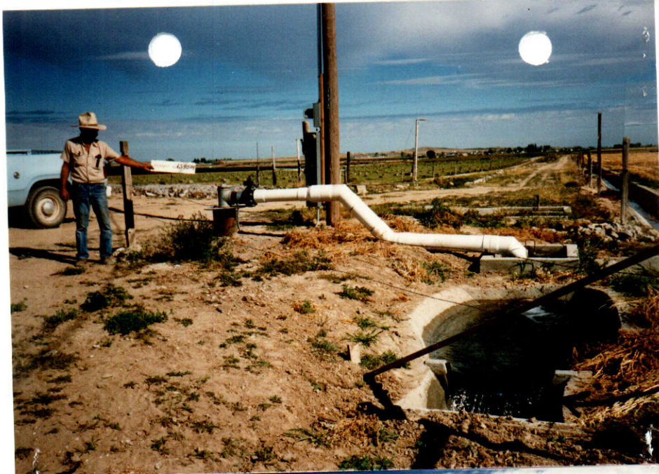
LOOKING NORTH P/D 2' WEIR
